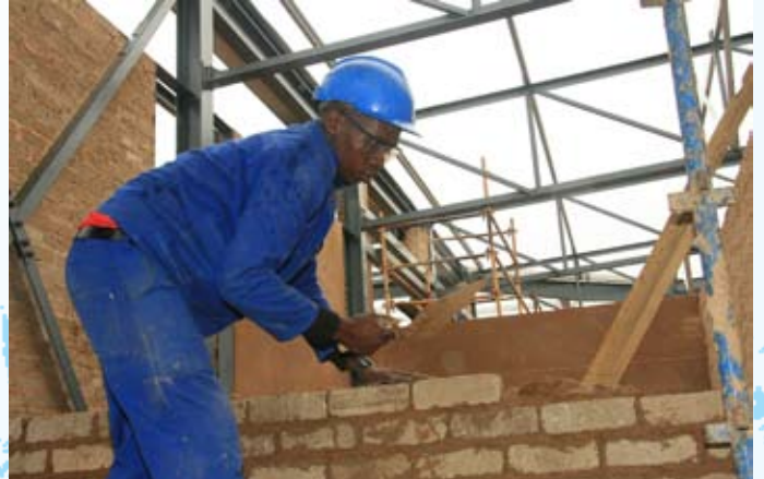
A project undertaken by the Ugu Emerging contractors
