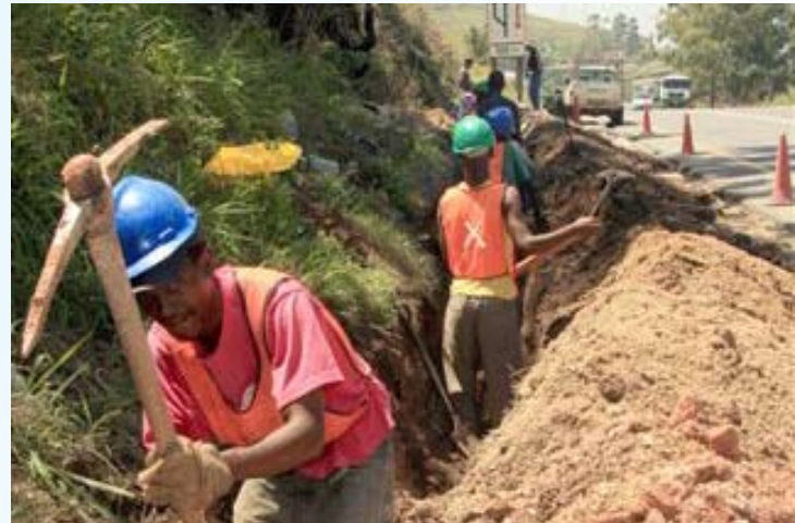
South Coast Bulk Pipeline
